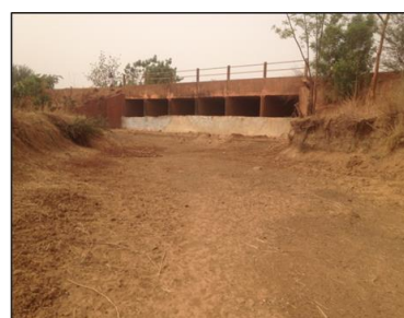
A wall built under a bridge in Lawra to retain water
