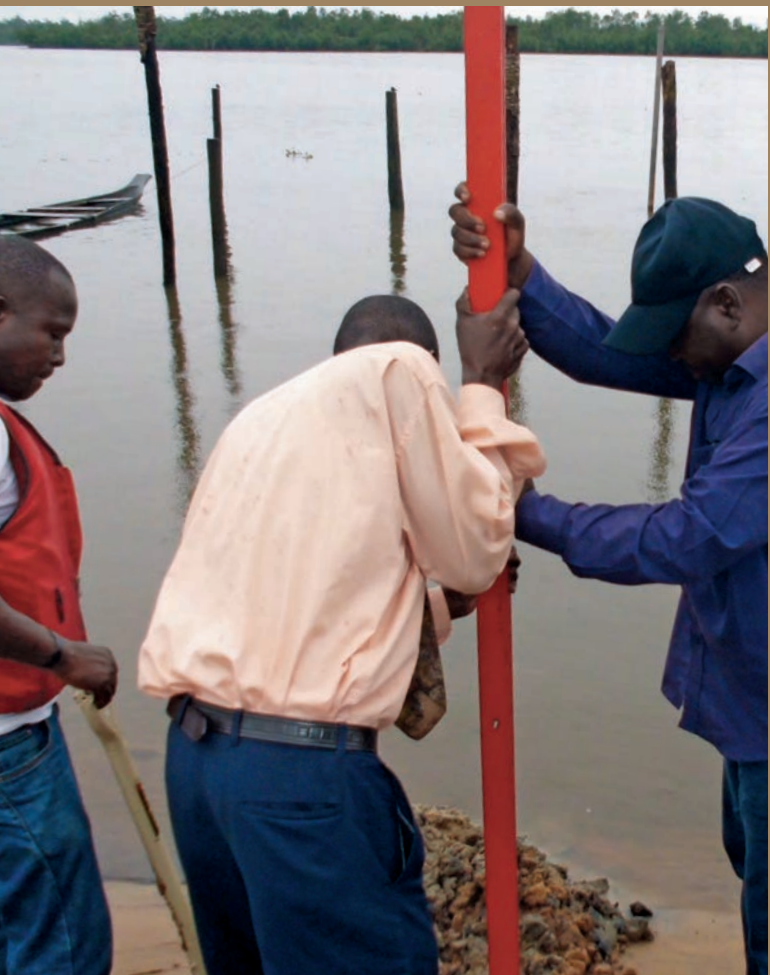
Researchers assist in installing flood gauges.
