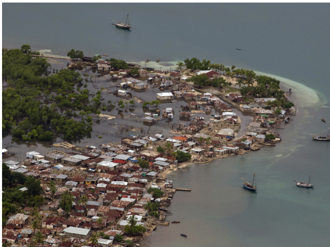
Hurricane Sandy inflicts heavy damage in Haiti Source: UN
