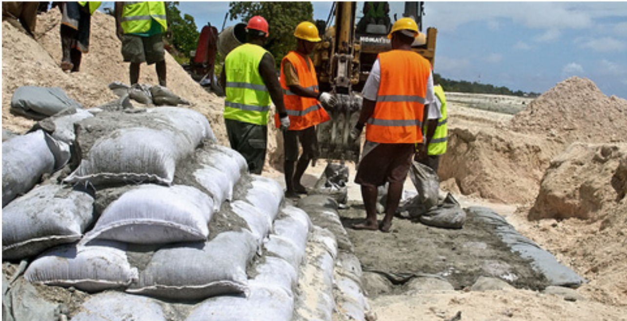
Building a sea wall in Kiribati Source: World Bank
