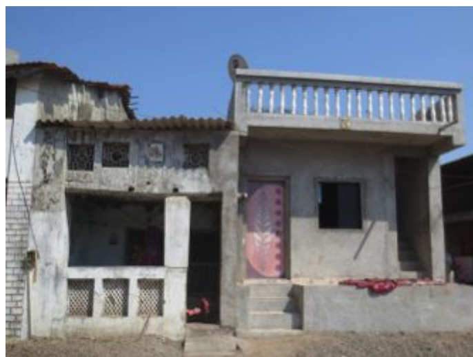
Photograph 5: A newly constructed house with raised plinth and terrace (yet to be completed and occupied) adjacent to the older house affected by 2006 floods at Moti Ved
