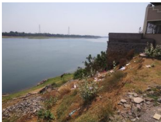
Photograph 13: A private river embankment, built from stone and concrete for INR 3.5 million, was destroyed during the 2006 flood at Abrama
