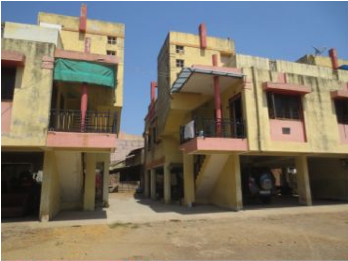
Photograph 7: Houses of brothers reconstructed after 1998 floods with only parking at the ground level, Bhesan village
